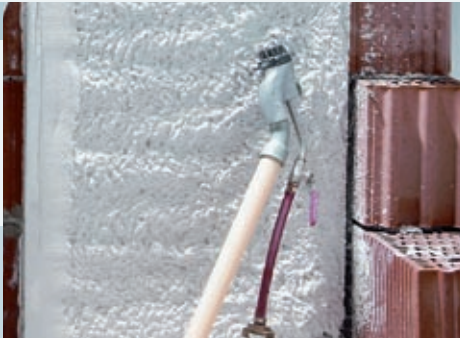
Figure 3: Spraying and the first even out after 5 minutes
