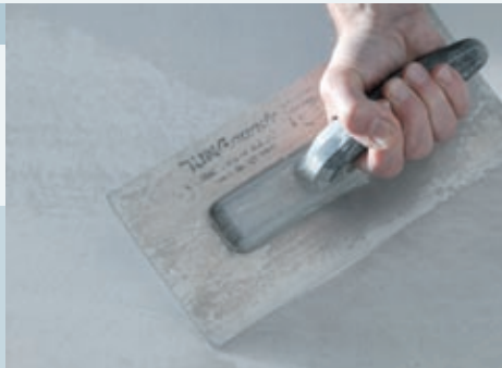
Figure 6: First smooth finishing after 150 min; sound velocity of 550 m/s
