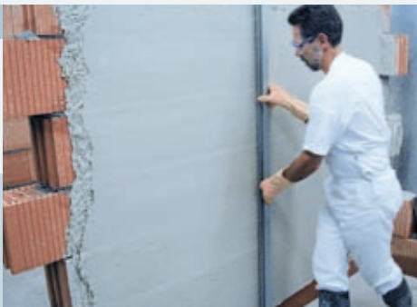
Figure 4: Paring of surface after 60 – 80 min corresponding to sound velocity of 125 m/s
