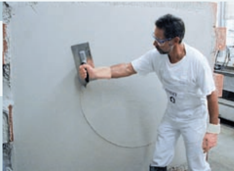
Figure 7: Last smooth finishing after 170 min; sound velocity of 650 m/s
