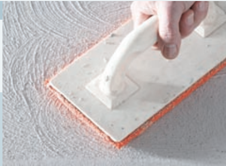
Figure 5: Rough finishing after 120 min corresponding to sound velocity of 300 m/s
